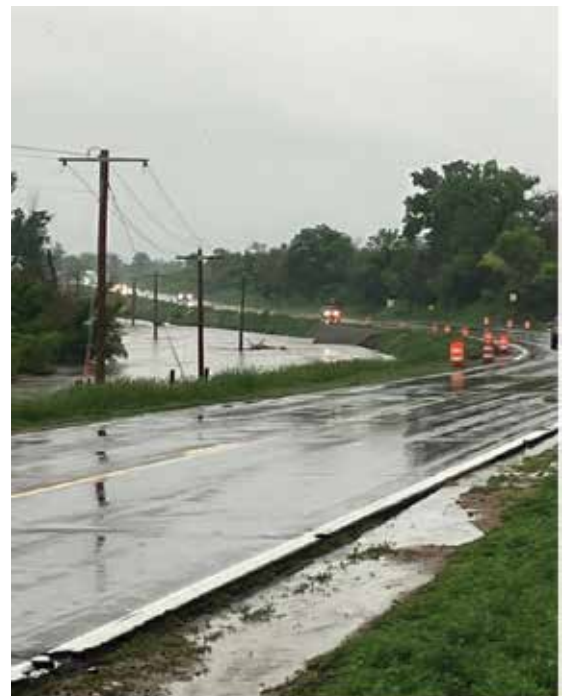
Flooding at Palisade on May 26th (12" of rain overnight).
